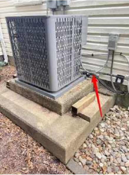
The L flashing would go up the wall a minimum of 4 inches and out onto the pad at least 2 inches. Then the base of it would be installed down over the top of the flashing and then the siding would be installed.
